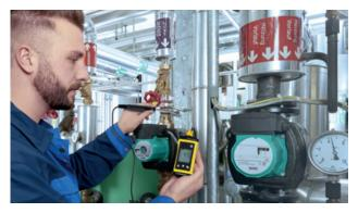
To operate in an energy-saving, comfortable and fail-safe manner, perfect adjustment, and function are crucial for heating systems. During commissioning and maintenance, temperature measurements, e.g. on supply/return temperatures, show whether the optimum operating condition is ensured. After hydraulic balancing sound heat distribution can be checked quickly and reliably with the G 1202.
